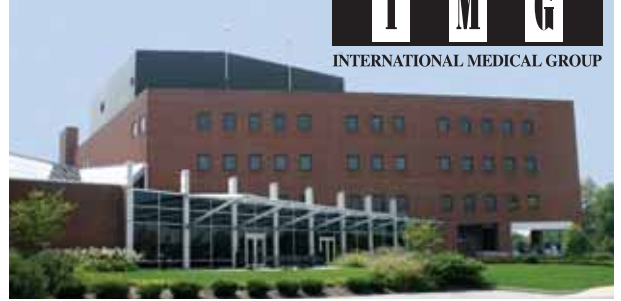
IMG World Headquarters, Indianapolis, Indiana
